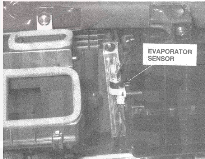
65. Behind Right Side of Dash (Dash Removed)
